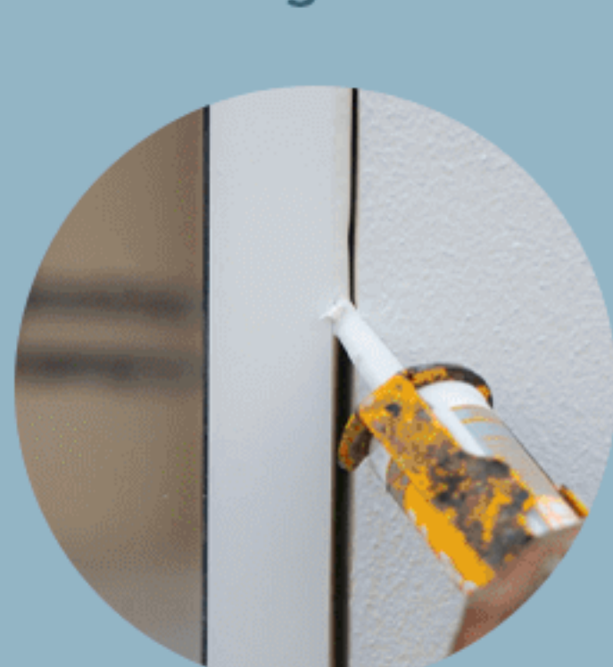
SEAL AROUND DOORS AND WINDOWS
